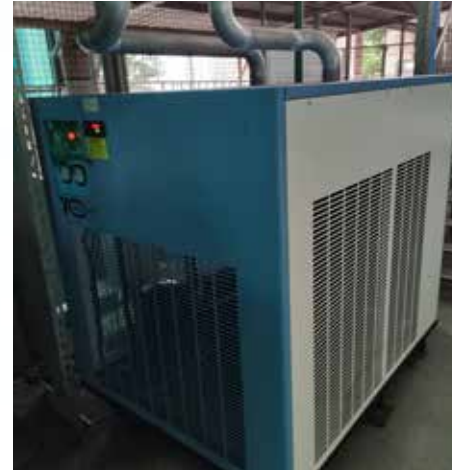
Replacing the old freezing dryer for a new one
