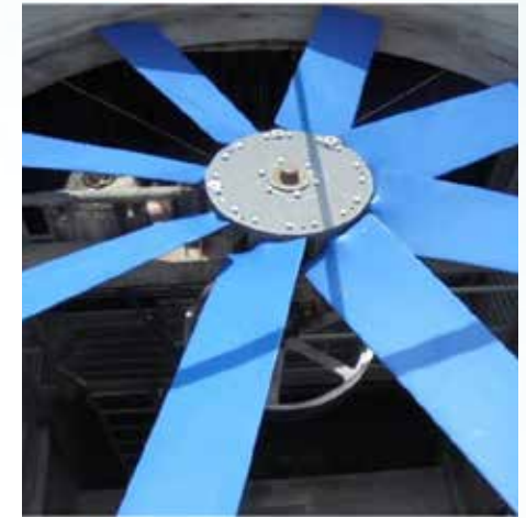
Replacing the aluminum fan blade to FRP energy conservation fan blade in the cooling tower
