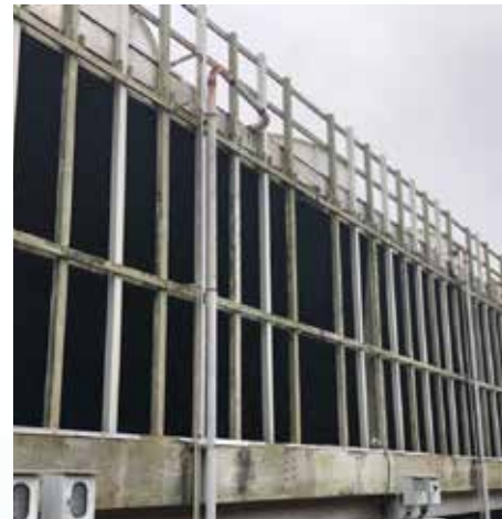
Replacement of fins and renovation on cooling water tower
