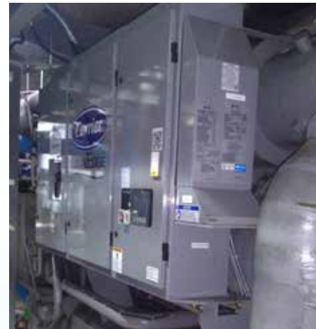
Replacing the variable frequency ice machine in AC1+AC2
